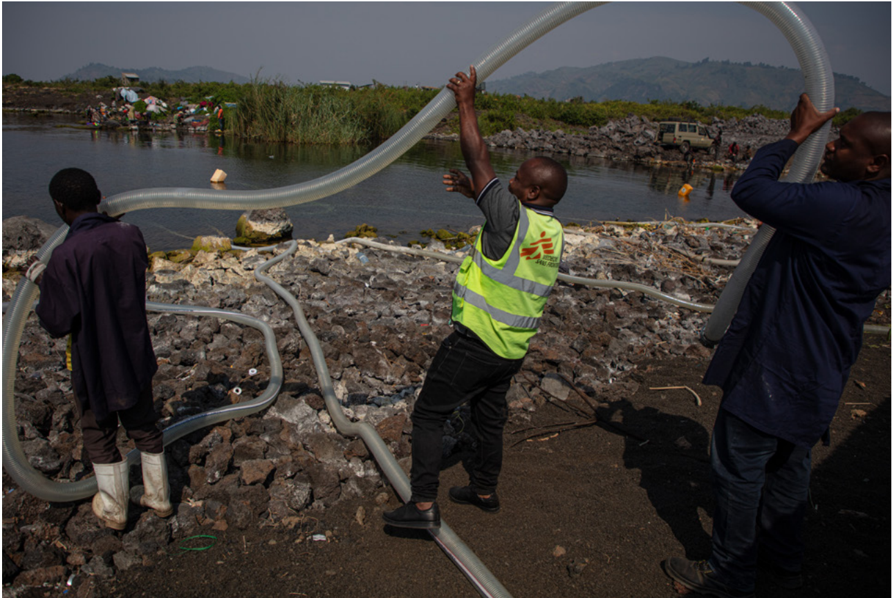
↑ MSF team conducts maintenance at Bulengo water treatment plant, pumping and treating Lake Kivu water with chlorine before distribution to the displaced camp tap network. Democratic Republic of Congo, July 2023. Photo: Alexandre Marcou/MSF
